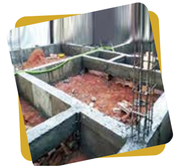
Basement Height – 2 Ft (from Existing Ground Level)
