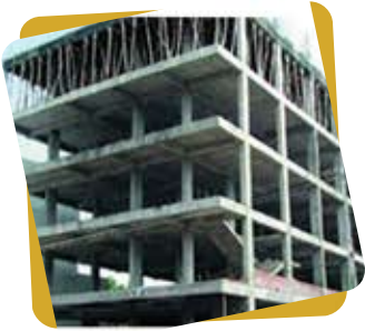
RCC Framed Structure
