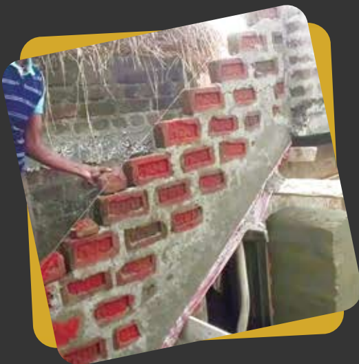
STAIRCASE Brick Wall
