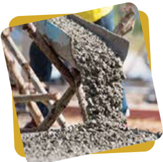
Concrete Grade M20 (Manual Mix)
