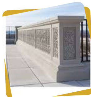
Parapet Wall – 3' Feet Height/ 4Inch Thick
