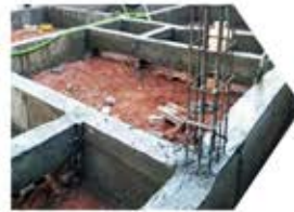
Basement Height – 3 Ft (from Existing Ground Level)
