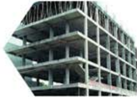
RCC Framed Structure as per Structural Drawing.
