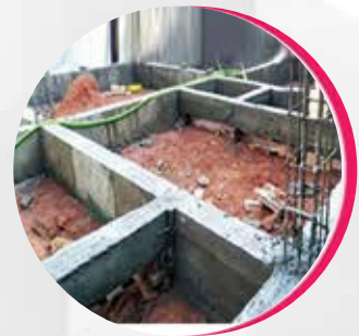
Basement Height – 3 Ft (from Existing Ground Level)
