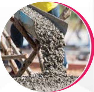
Concrete Grade M20 (Manual Mix)
