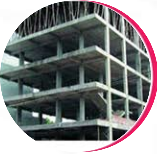
RCC Framed Structure
